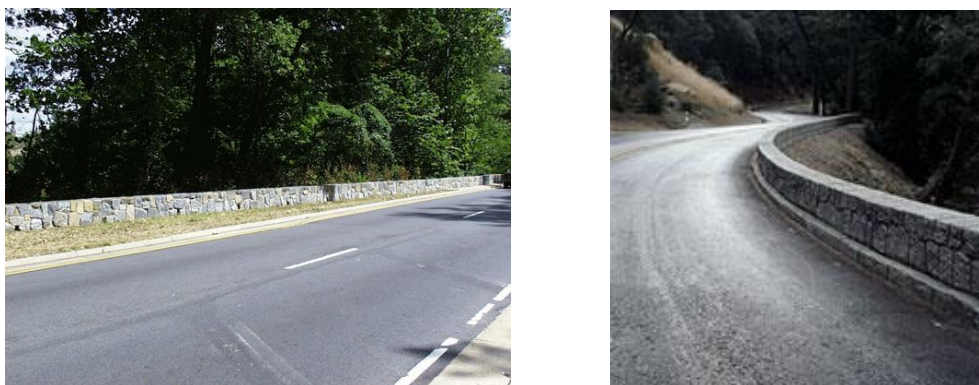
Figure 6-1: Typical examples of masonry guardwalls.
