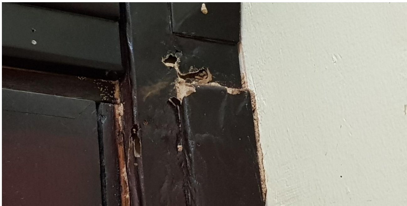
Subterranean termite damage on door frame
