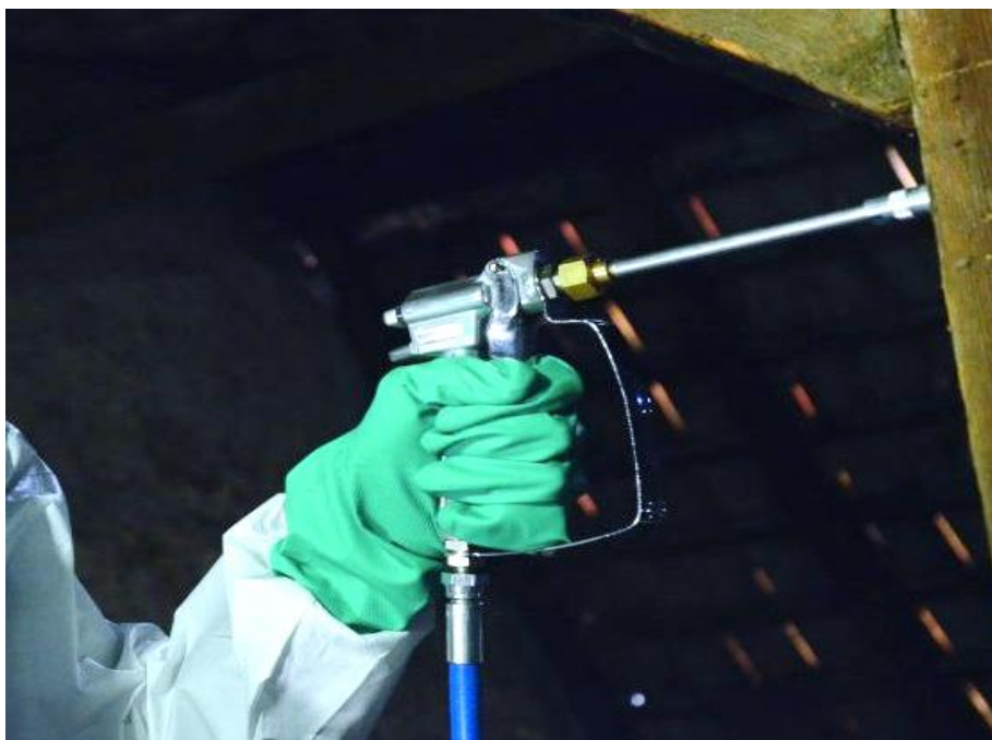
Injecting termiticides into drilled holes using termiticides injector
