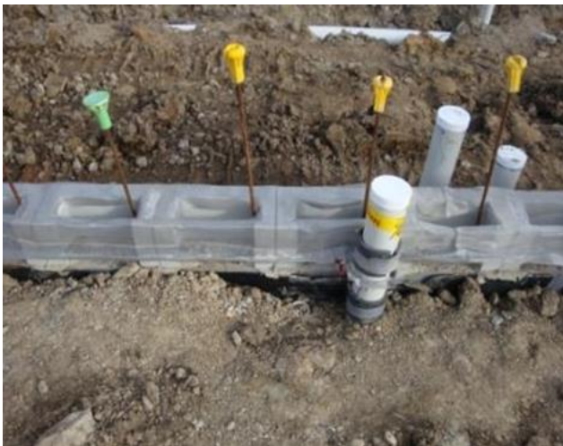
USE OF ANTI TERMITE MESH AROUND UTILITY PIPE PENETRATION
