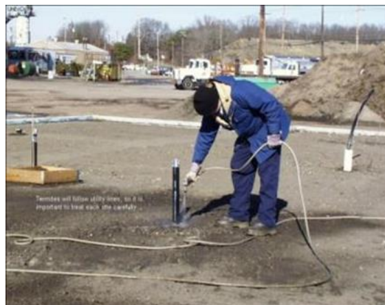
TYPICAL SECTION - ANTI TERMITE TREATMENT AROUND UTILITY PIPE PENETRATION
