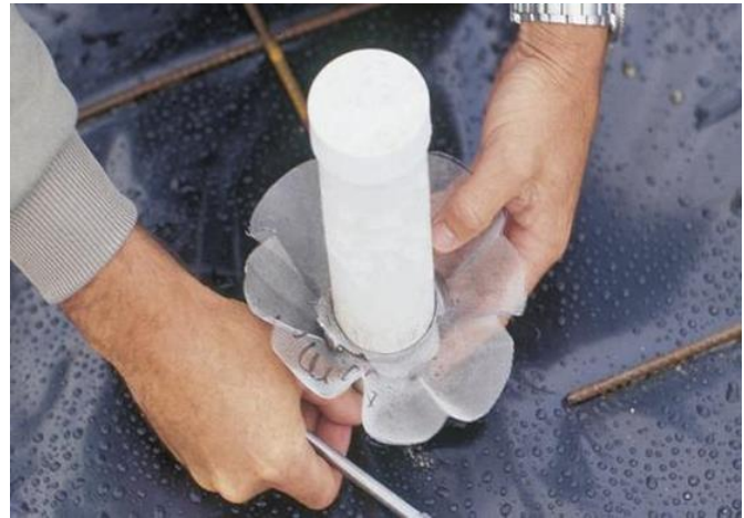
USE OF ANTI TERMITE MESH AROUND UTILITY PIPE PENETRATION
