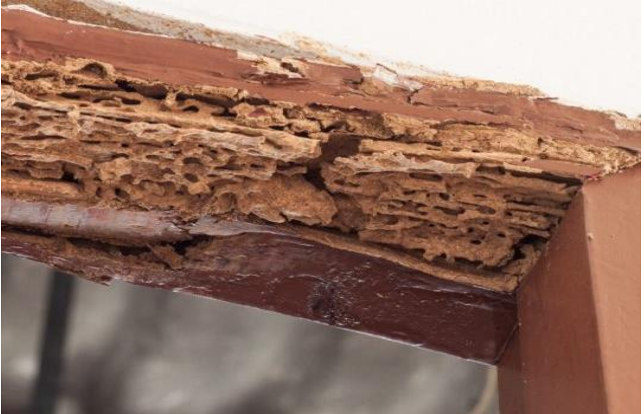
Subterranean termite damage on wooden structures
