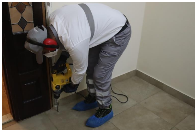
Drilling ground holes
