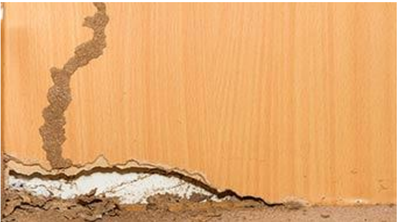
Subterranean termite damage on door frame
