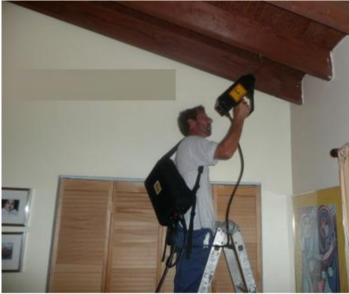
Dry wood electrocution treatment using electrogun
