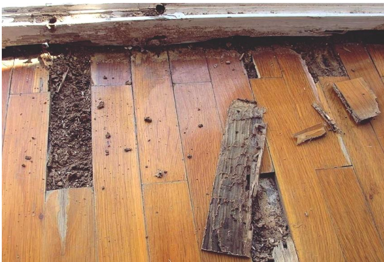
Subterranean termite damage on hardwood floor
